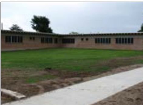
The Winters Dorm replacement building dorm will begin construction next year.
