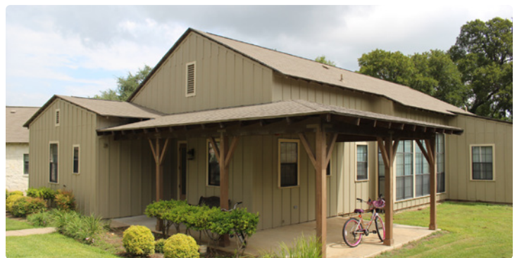
Above: Various stages of construction for the newest Cottage at The Village. Bottom Picture: What the new Cottage will look like upon completion.
